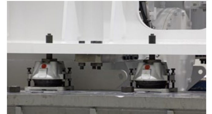
Structure-borne noise levels measurement below soft elastic mount
